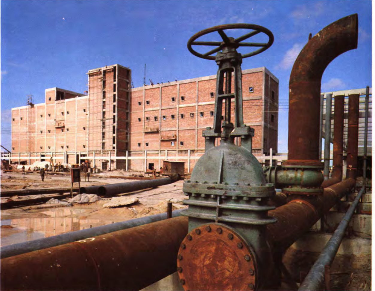
COBAFI Companhia Bahiana de Fibras S.A., a 45% Akzo participation, will commence operations in its nylon tire-reinforcing materials facility at Salvador (Brazil) in the middle of 1978.
